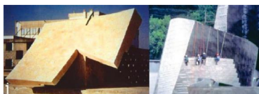
Figure 7. 1:1 Mockup That Assembled on The Site Source: Lim, 2010
