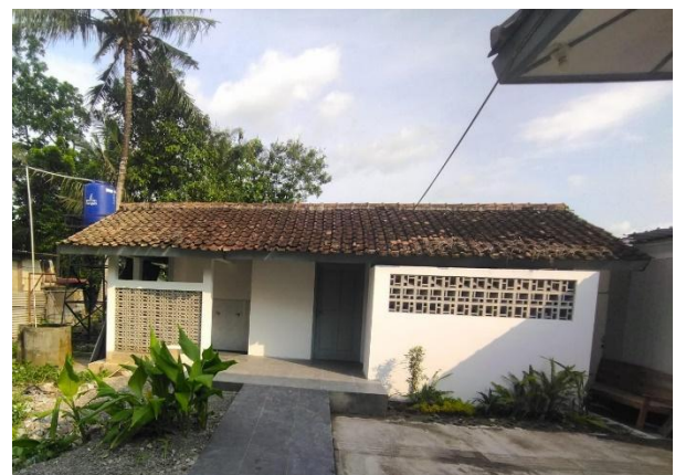
Gambar 6. Tahap Finishing Toilet
