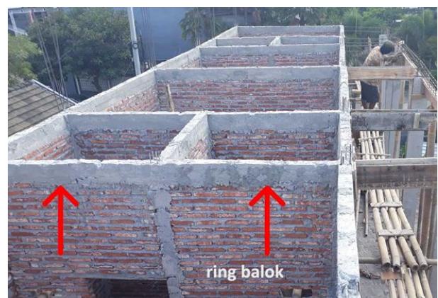
Gambar 7. Balok Ring [11]
