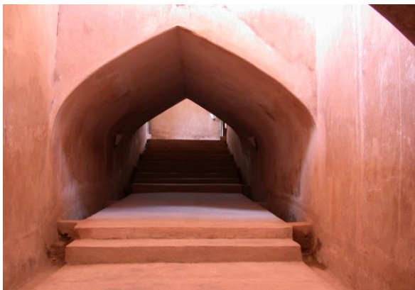
Figure-6: Aisle with a distinctive arch on the Sumur Gumuling in Tamansari (Source: collection, July 5, 2005)
