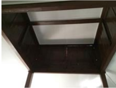
Fig. 13: View to the wooden panels and 'dada peksi' main beams in Jangkang Mosque (source: Survey images)
