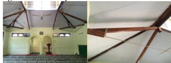
Fig. 17: Mosque in Sudimoro (left: sacred area, right: structure of hanging tajug roof) (source: Survey images)
