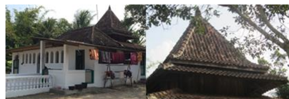
Fig. 12: Mosque in Jangkang (left: exterior, right: tajug roof) (source: Survey images)
