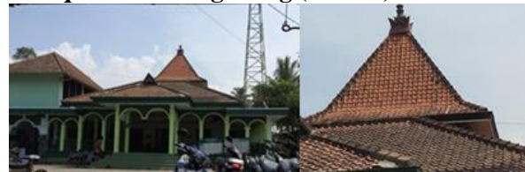
Fig. 8: Kyai Raden Santri Mosque (left: exterior, right: tajug roof with iron sheet crowning on top) (source: Survey images)
