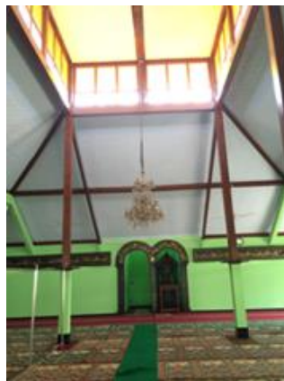
Fig. 9: The soko guru and top windows (source: Survey images)
